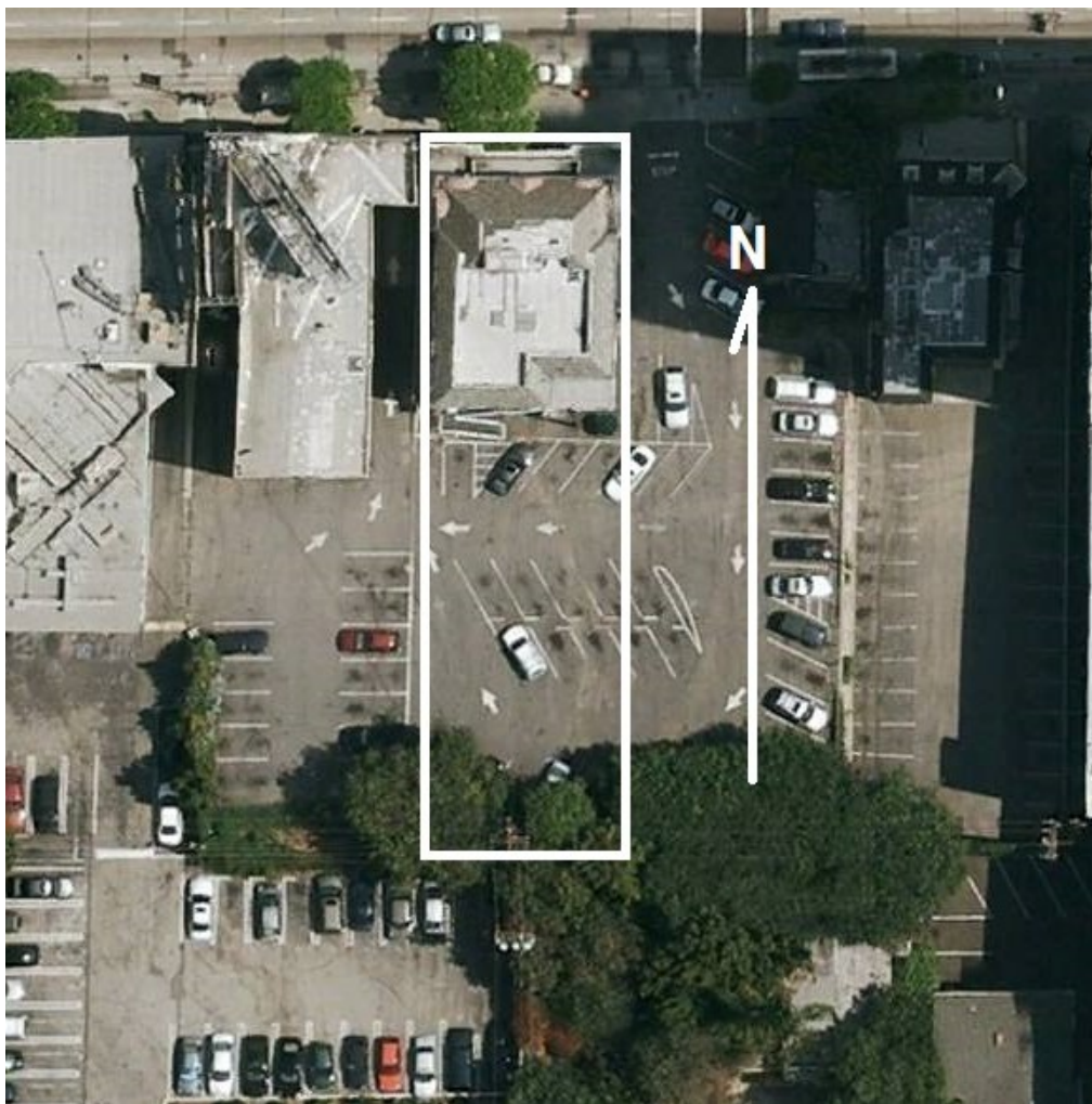
Photograph from Google Earth (7 October 2007) Building Center: 34.090385 N 118.388667 W
